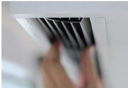
You can turn the air discharge element easily by hand up to 16 degrees towards the in- or outside. So that you obtain maximum insulation, the air discharge element must be turned appropriately towards the outside.
